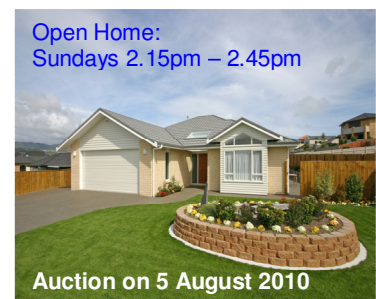
342 Manly Street Paraparaumu Beach
